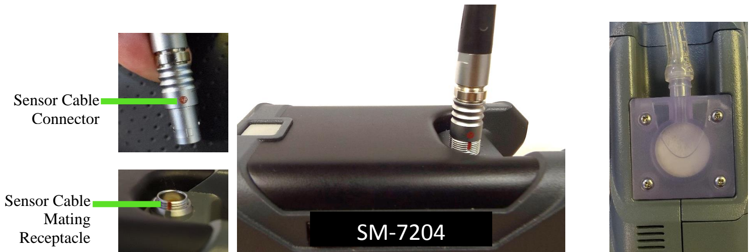
Figure 3-1. Sensor Cable being connected to SM-7204 and tubing connected to air intake
